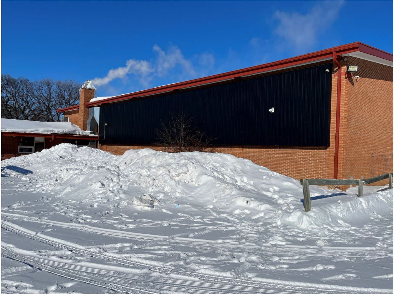
There is a solar wall that helps heat the gymnasium – will be utilized with the HVAC renovation.
