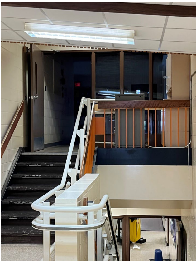
Despite being built in an era when accessibility was rarely considered the school faced the challenge by installing a chair lift that allows accessibility to 3 floors.
