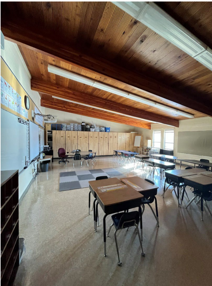
Classrooms from the 1982 addition.
