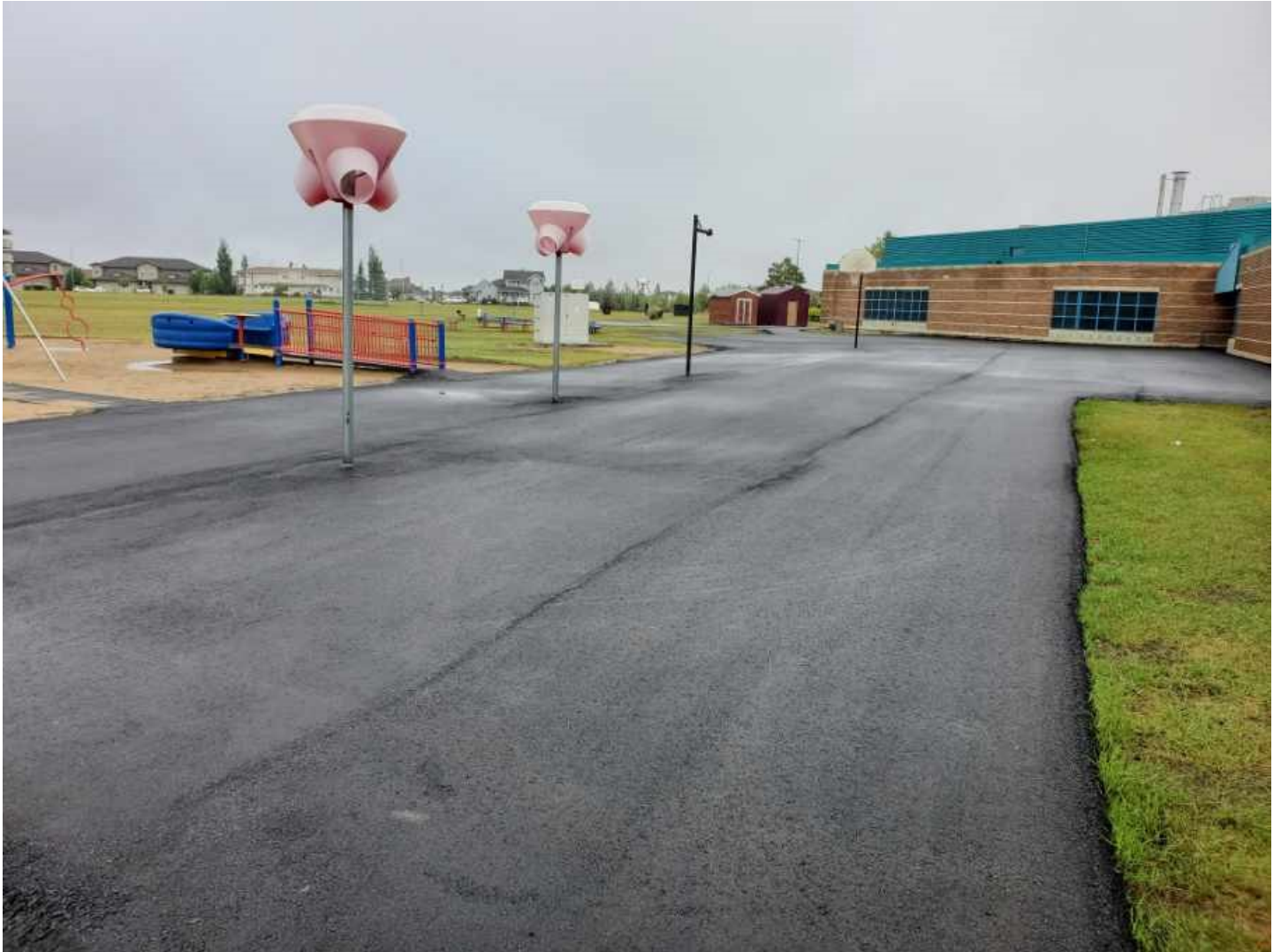
MC Knoll Drainage and Settlement Repair - Asphalt
