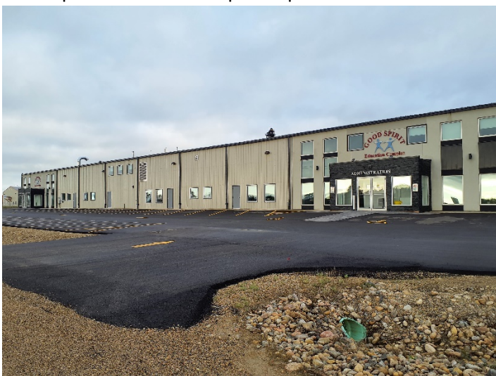
Good Spirit Education Complex Asphalt and Patio
