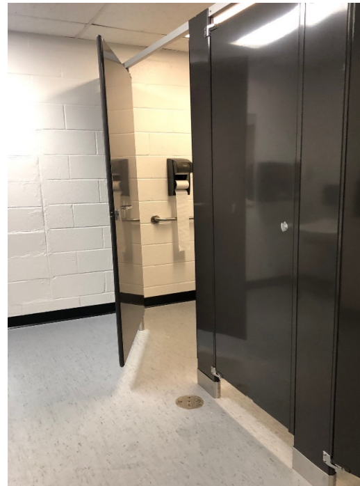
Churchbridge School Washroom Reno
