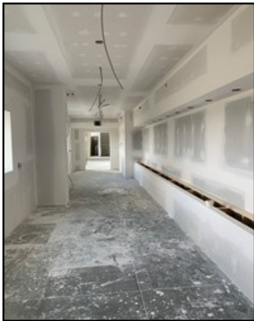
Photo above: Connecting hallway between Phase I and Phase II .
