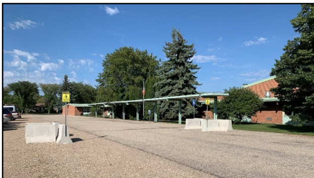
Photo above: A cross walk was created using jersey barriers.
