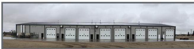
Photo above: Bus garage area at the new facility
