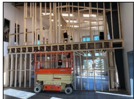
Photo above: The GSEC gets new walls!
