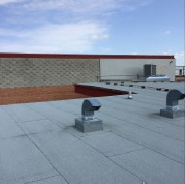
Sturgis Brick Repairs
