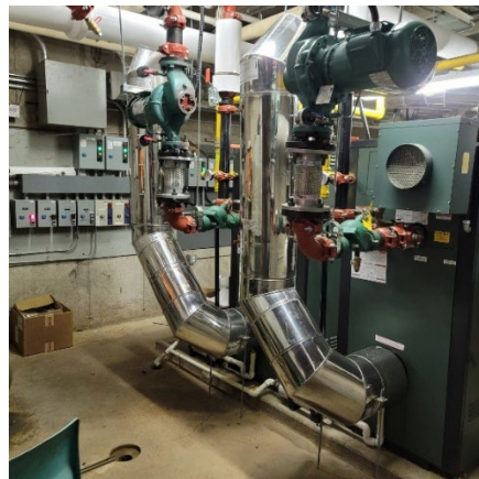
KCI Boiler Replacement
