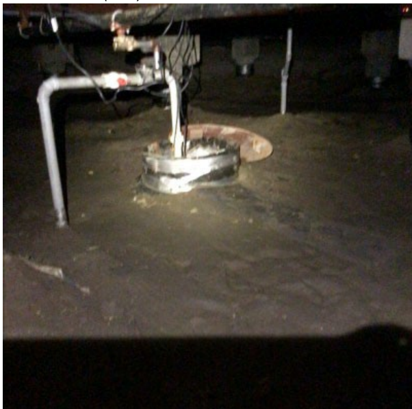
Crawlspace under Portables
