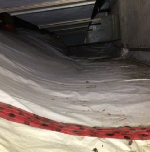
Crawlspaces and Boiler Room:
