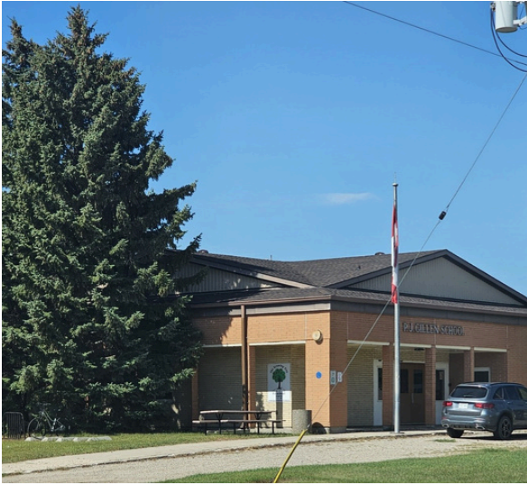
Shingles were replaced over the office area at P.J. Gillen School.
