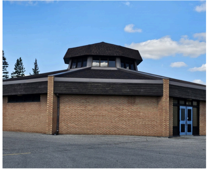
Shingles were replaced over the student center at Yorkdale Central School.
